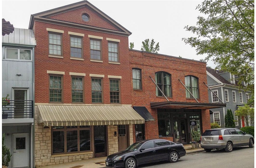
Live-Work Building Palmetto, GA
