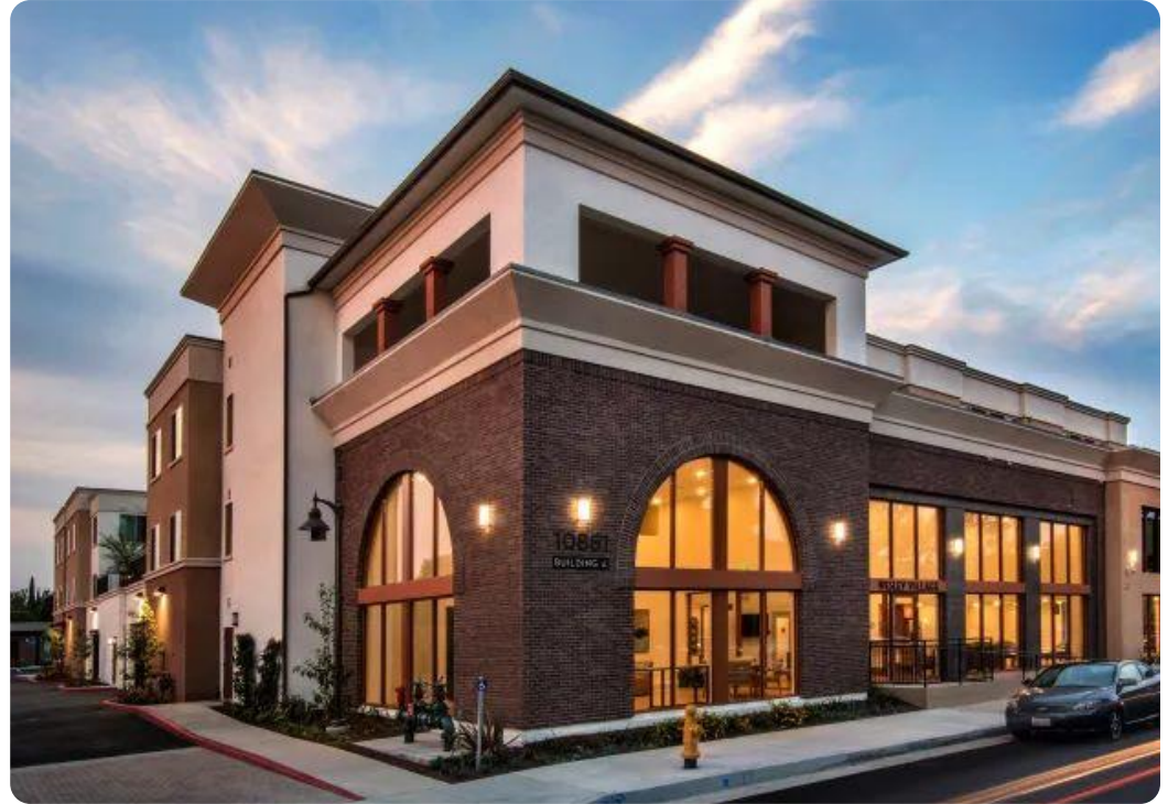
Wesley Village Affordable & Senior Housing Garden Grove United Methodist Church. Garden Grove, CA
