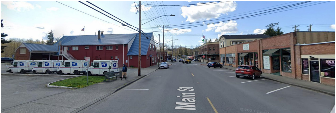
Figure 13 Existing Development along Main Street
